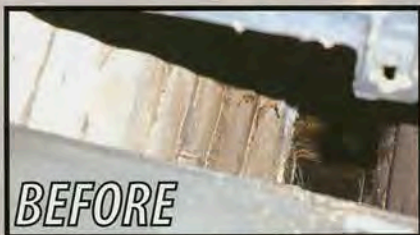
Exposed Brick Corbells Before HeatShield Cerfractory Foam
